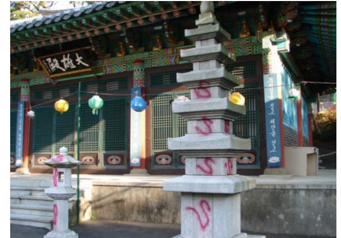
Vandalized structures in Gaeunsa Temple, Busan, one of many such cases.
